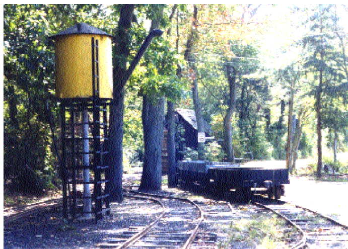
Fueling facilities with two low-sided flatcars used for hauling baggage
