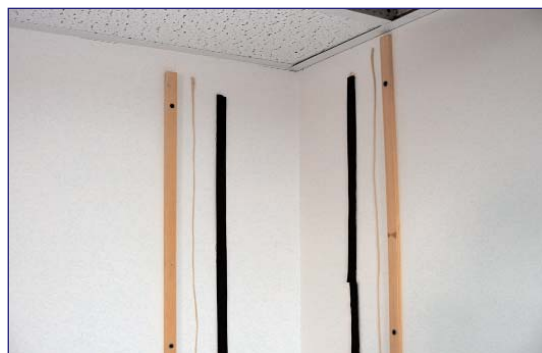
Velcro strips in place with bead of Liquid Nails
