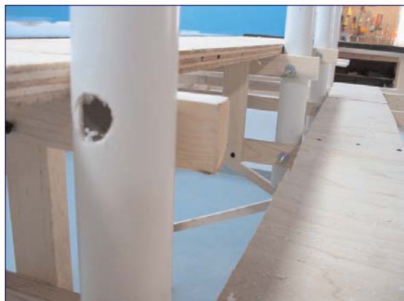
PVC pipes bolted to benchwork
