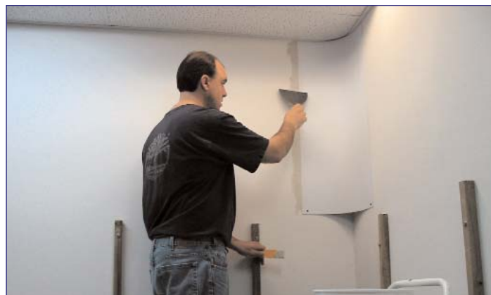
Applying drywall joint compound
