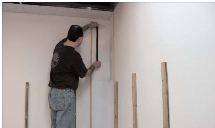
Applying the Velcro strips
