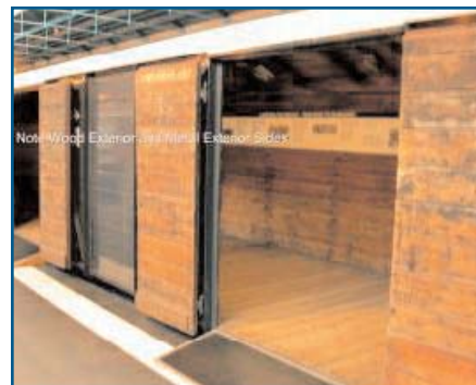
Figure 4: Note the doors on this box car.
