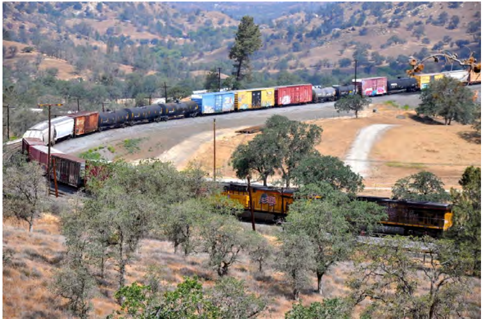
The lead end of a UP mixed freight headed upgrade (eastbound). The engines have already passed over the loop tunnel and are about to exit the loop area and head into Tunnel #10
