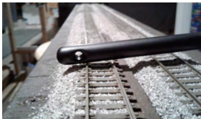
Tamping the ballast into place
