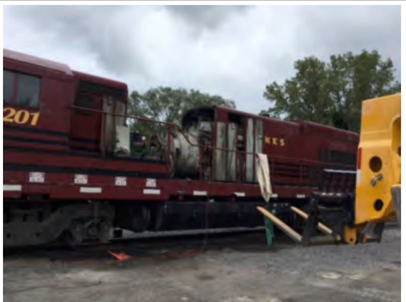
CORY On-The-Road Generator Replacement Project at Finger Lakes Railroad Facility
