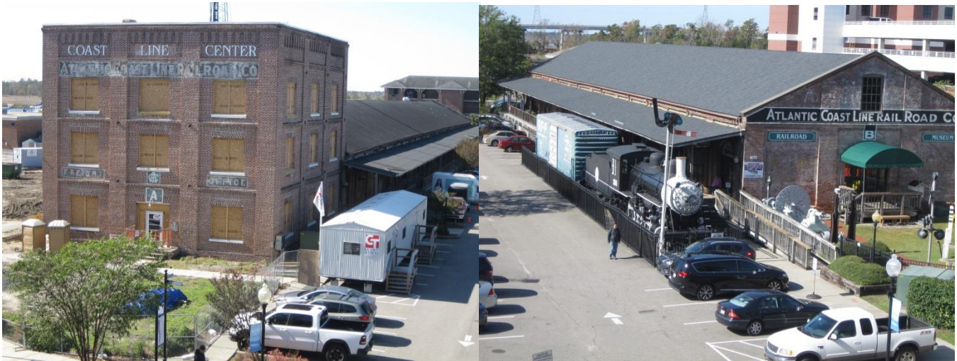
Warehouse A from the CFCC Parking structure Warehouse B from the CFCC Parking structure
