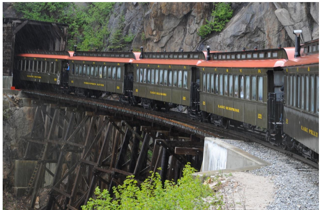
Fig 7. Exiting the original tunnel at MP 16, elev. 2275 ft.
