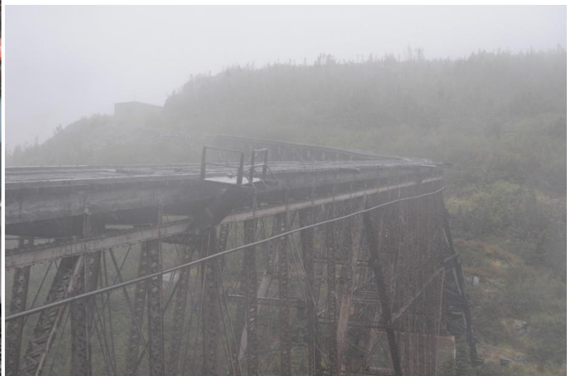
Fig 5. Abandoned bridge at Dead Horse Gulch, elev. 2613 ft
