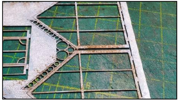
Photo 4: Closeup of rust effect
