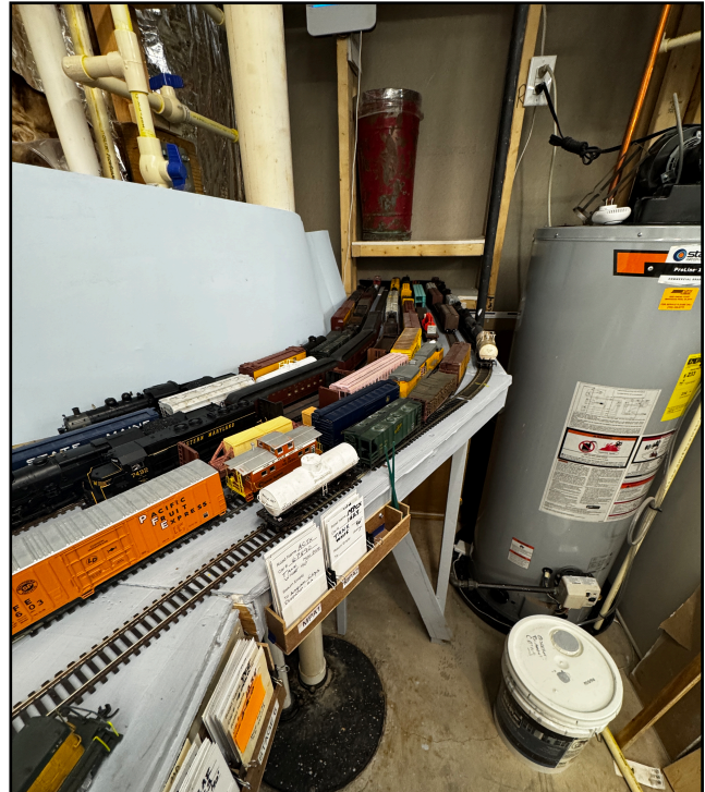
Photo 6: A closer view of the newly installed staging yard. The house utilities are accessible with the removal of two bolts, the staging section can be removed as a whole unit. Of course, this is after pulling all the rolling stock out of the yard....
