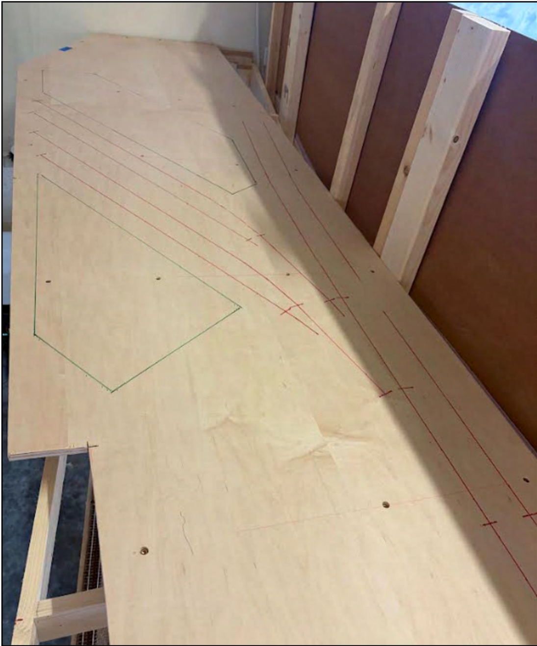
Photo 6 – Track and key structure locations indicated with permanent markers.
