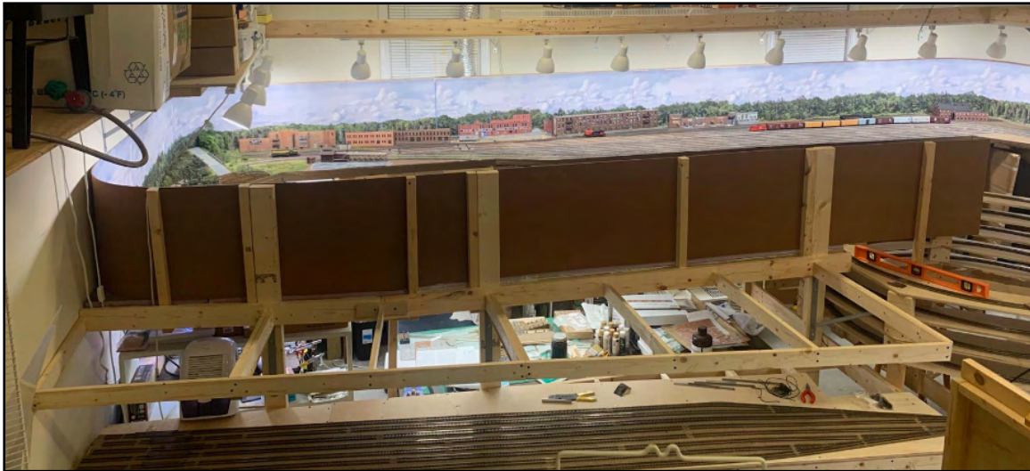
Photo 2 - Basic frame of open box benchwork mounted to shelf brackets on the back of the peninsula, above a staging yard.
